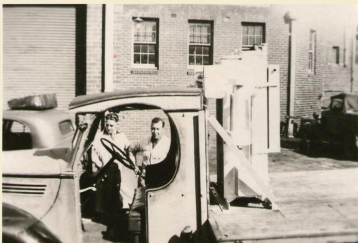
A gas producer attached to the tray of a Department of the Interior truck in Canberra. Photo: Jack Benson.
