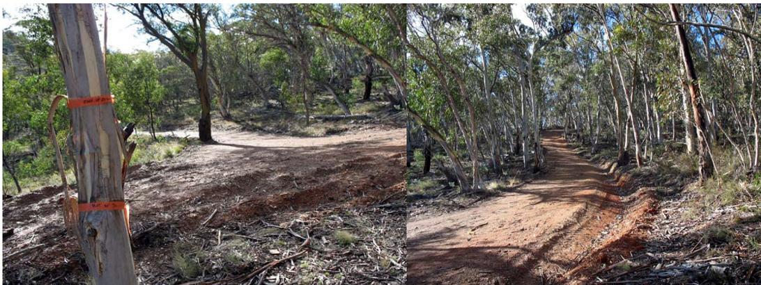
The current Mt Clear to Long Flat trail at the point where the Burnt Hill trail would join – note that the current trail is 4m wide but does not have the 2m shoulders.
