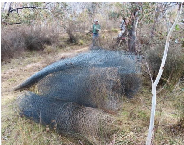
Fence removal. Photo by Brian Slee
